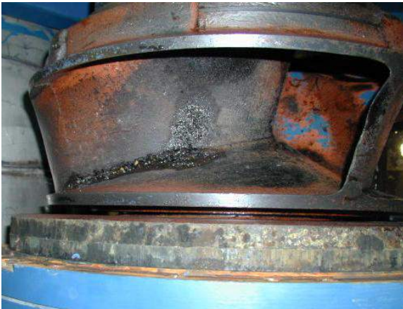
Erosion on pressure side
