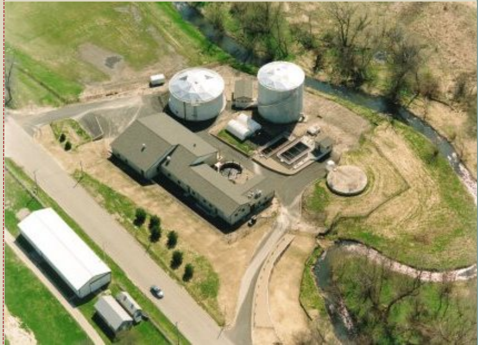
WWTF Aerial Photo
