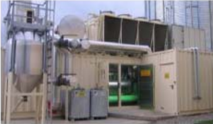
1 x containerized J420 fueled with biogas at Kogel, Germany
