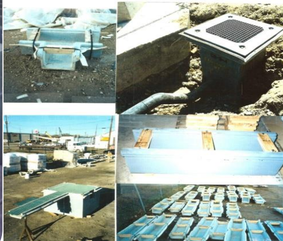
Precast Polymer Concrete Trench & Sumps Installation: Union Carbide and Phelps Dodge.
