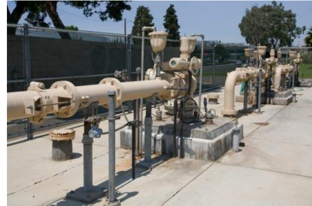
Typical injection well - OCWD
