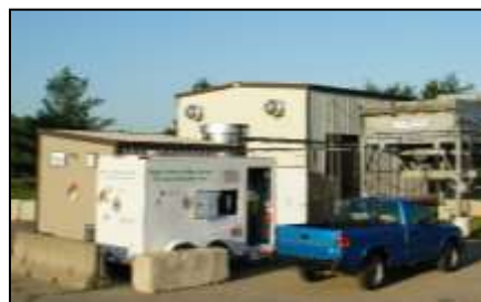
Temporary Fueling Station
