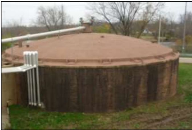
Waukesha WWTP Digester No. 4
