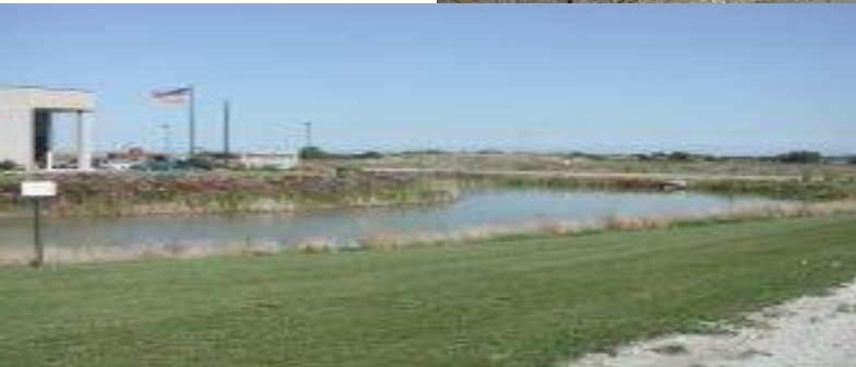
Wet Pond at Commercial Site – DNR photo
