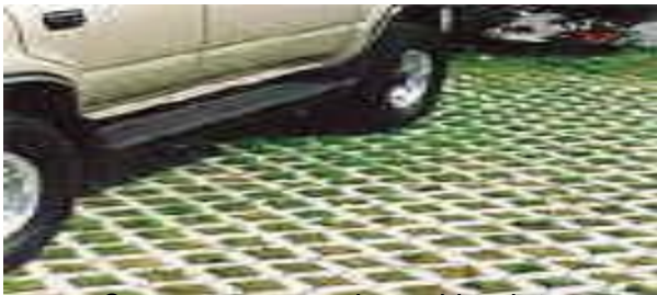
Concrete pavers in parking lot– DNR photo
