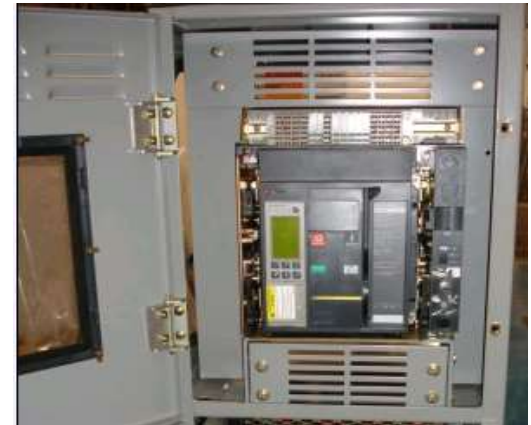
Completed Retrofill installation: front-view
