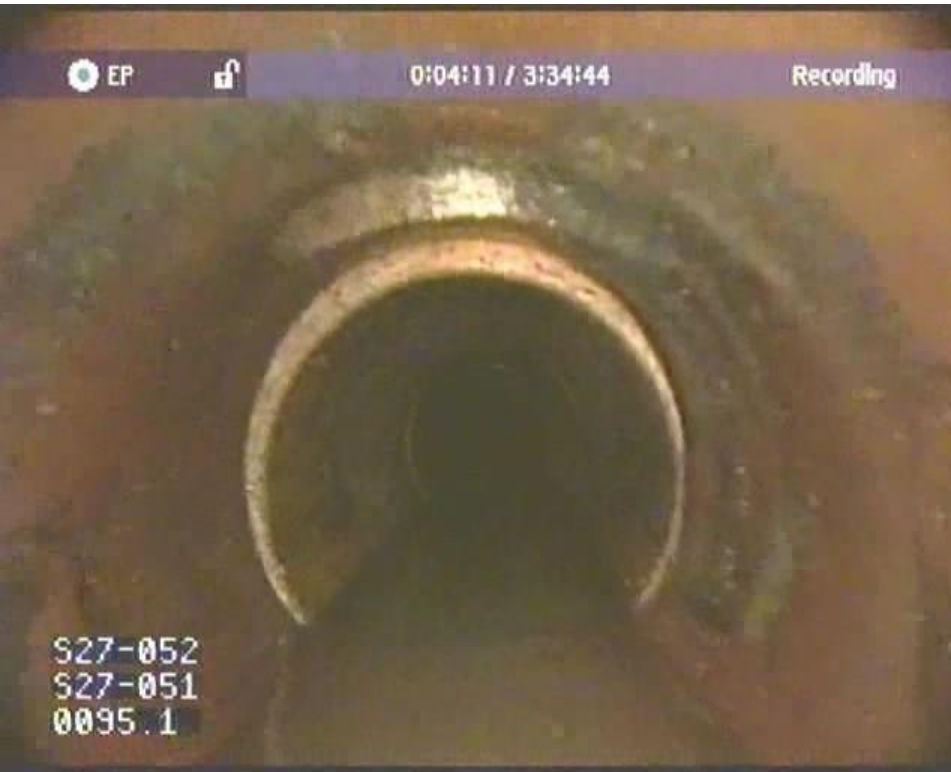
Sewer main & lateral connection prior to dye flooding
