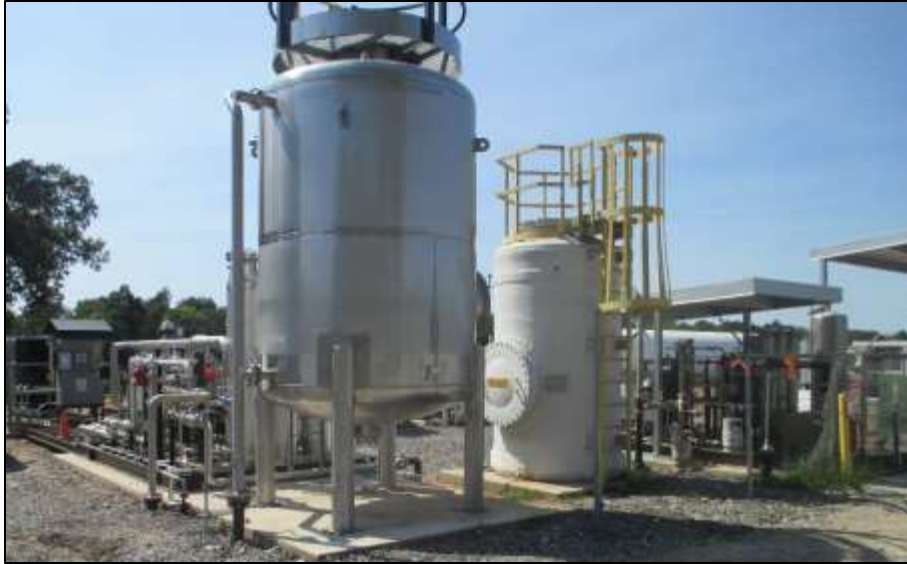
St. Landry Solid Waste, LA 1 – 50 scfm & 1 – 100 scfm BioCNG system
