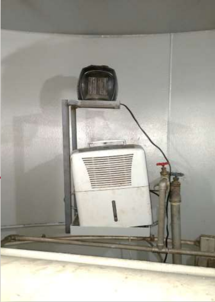
“Safety – From design to prototype. Heater stand platform at lift stations. Keeps the ceramic heaters in a safe spot.”
