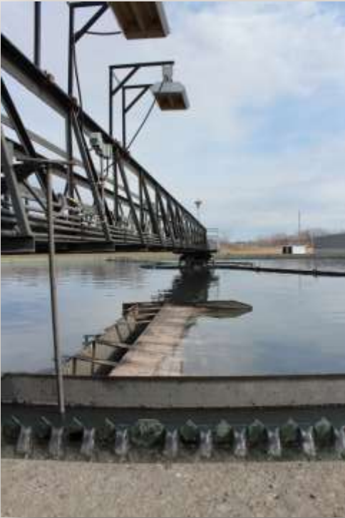
2017 Infrared Heaters – Waterloo, IA
