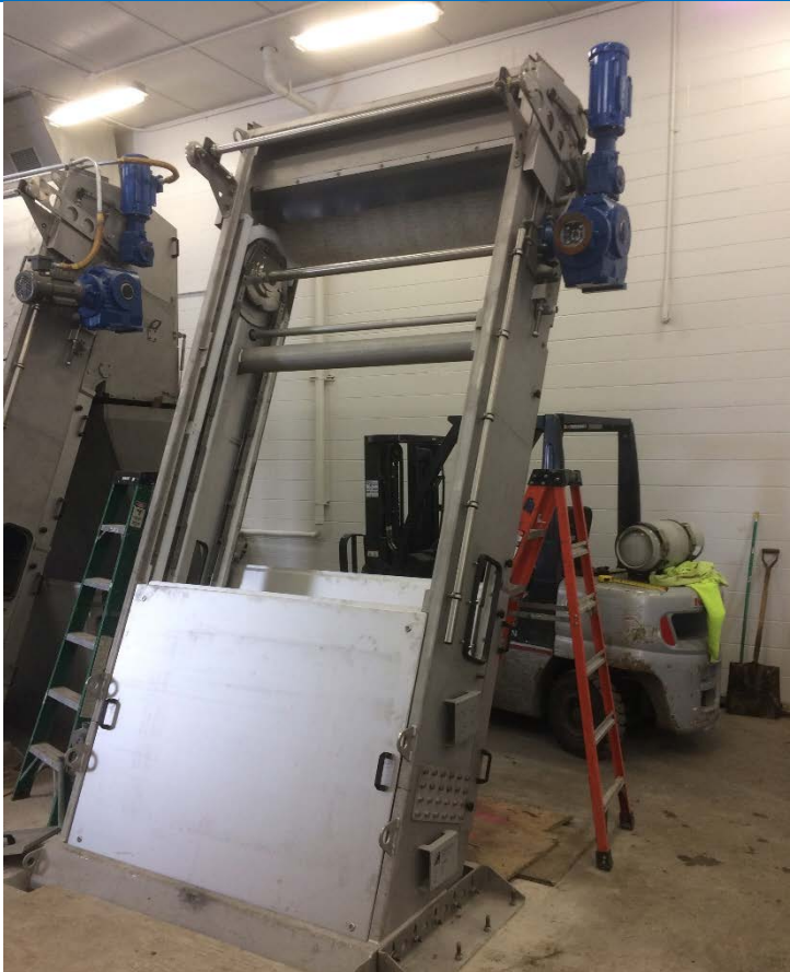
Screen installed without panels
