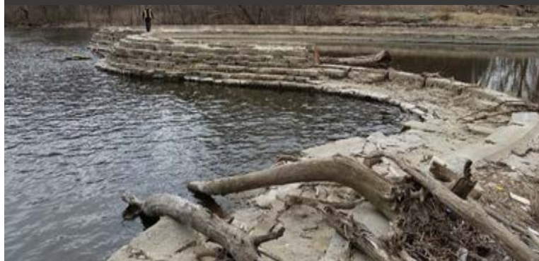
Water Resources Engineering
