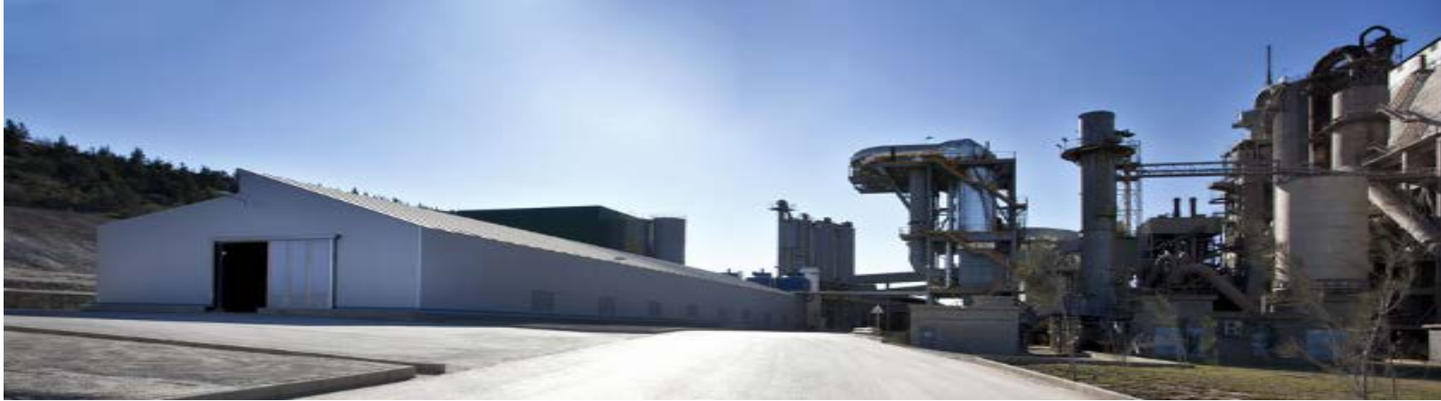
Site overview. The drying building is placed on the left whereas the cement plant is displayed on the right
