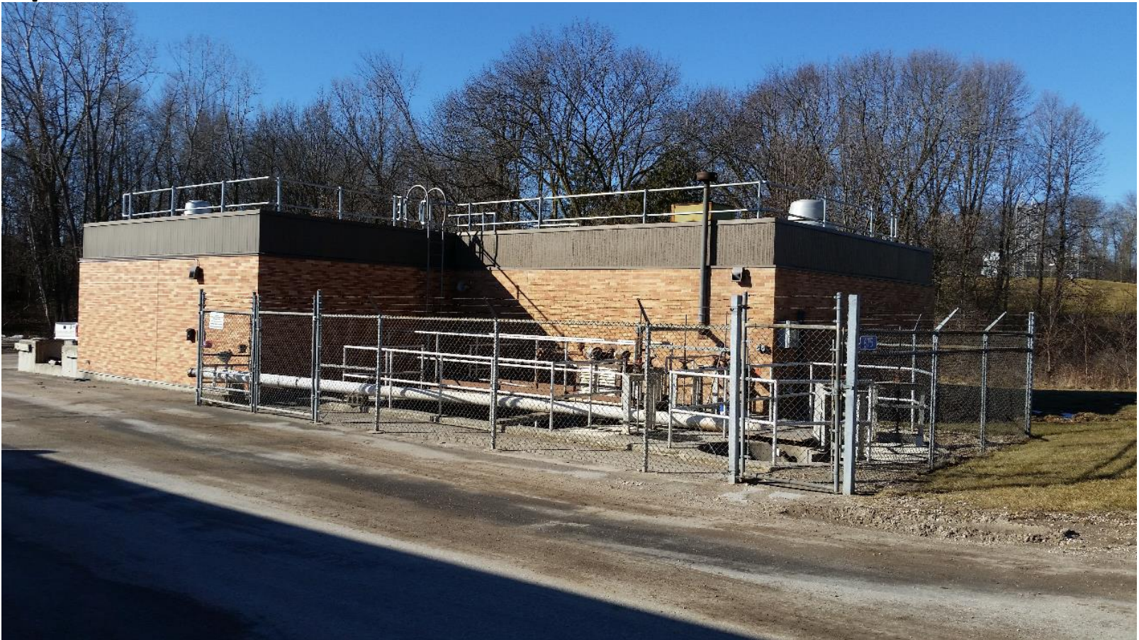
Fixed Ladder and Guardrail
