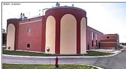
Madison Wastewater Treatment Plant Photo credit: Danielle Luke, Wisconsin DNR
