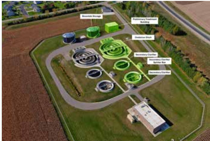
Figure 3 Site layout. Green highlights indicate locations for potential future expansion capacity.
