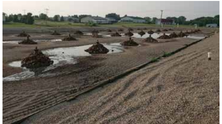
Figure 1 Recirculating sand filter facility (former plant)
