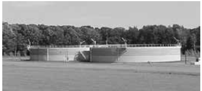
Biosolids storage tanks
