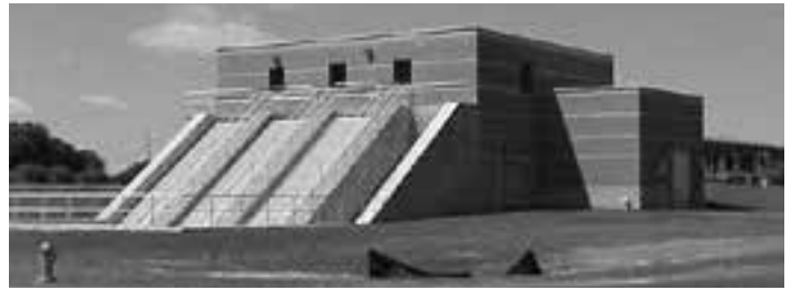
Influent pump station
