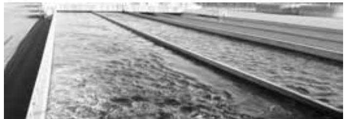
Oxidation ditches
