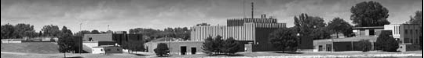
City of De Pere Wastewater Treatment Plant HST Integral Compressors
