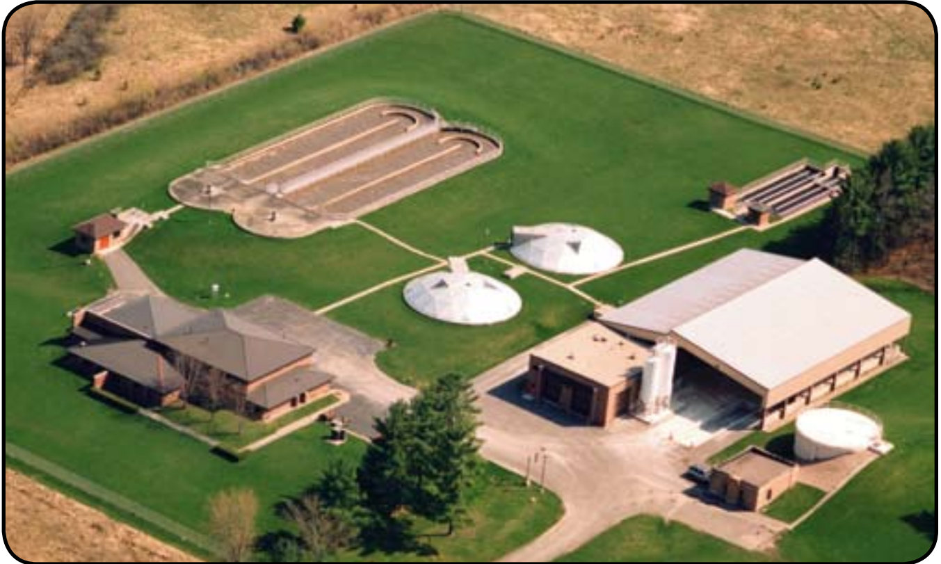
Baraboo Wastewater Treatment Plant
