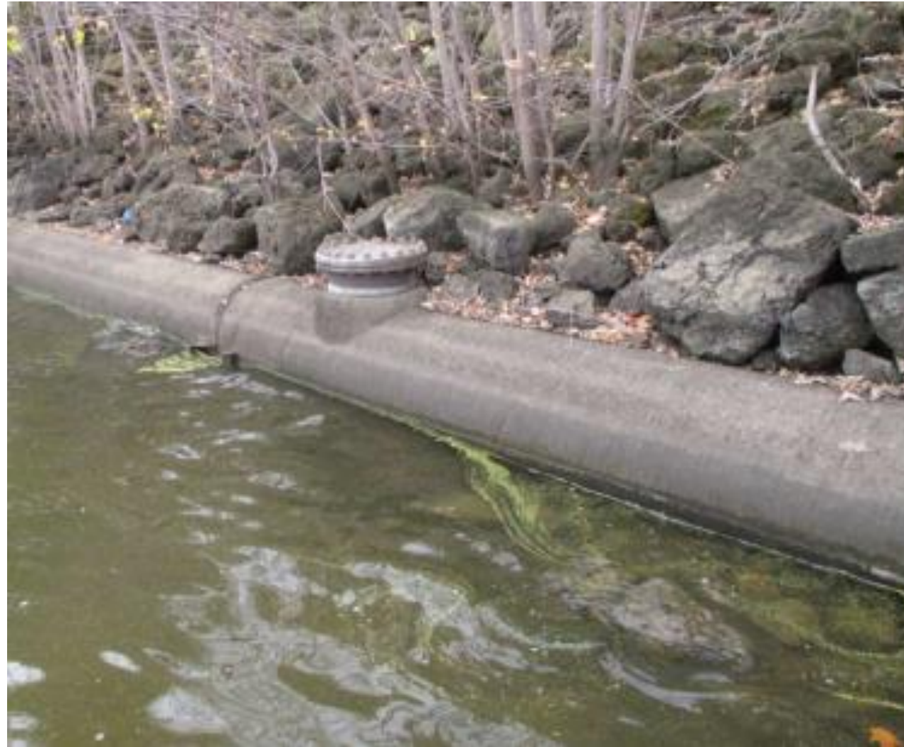
Courtesy of Strand Associates, Inc.
