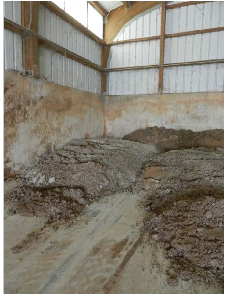
Significant Reduction in Stack Height
