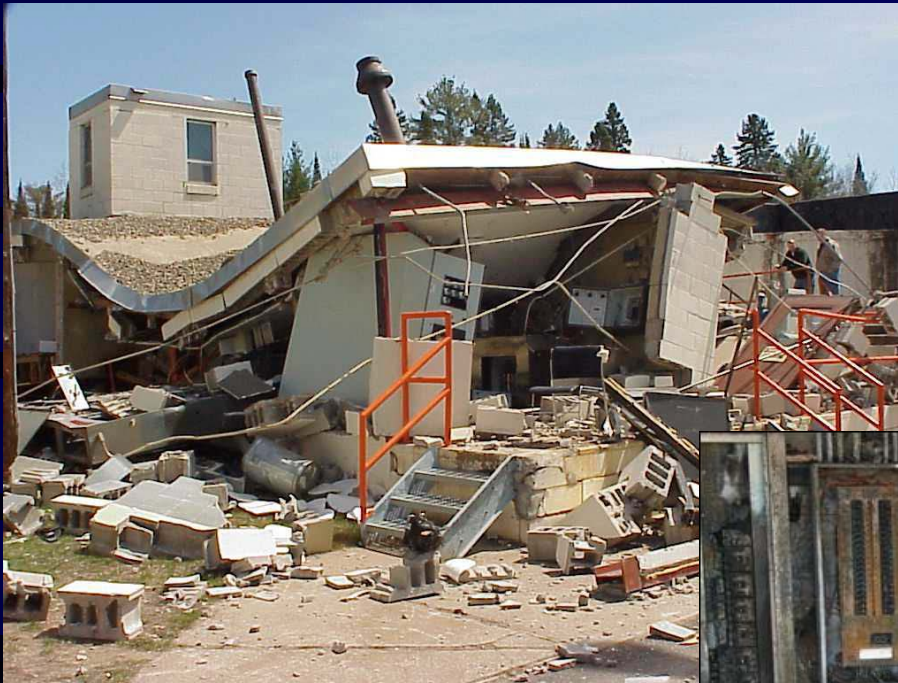
Main Control Building
