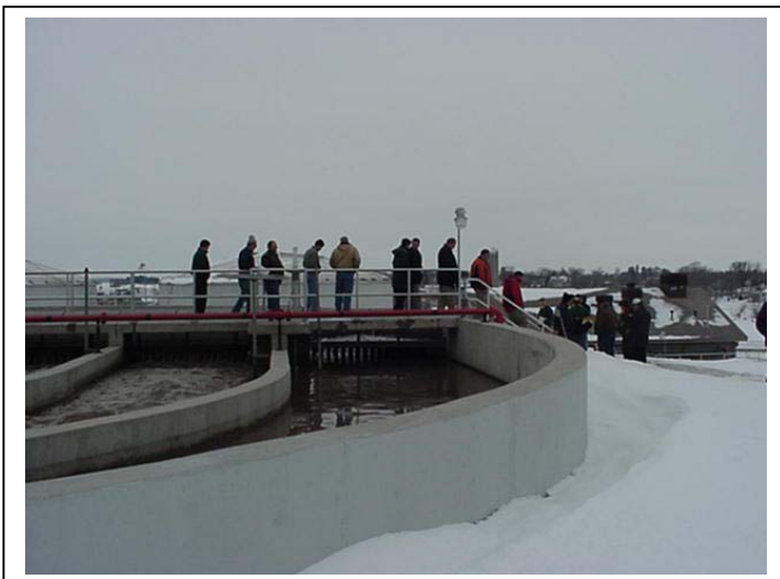
Operators inspect oxidation ditch at Marshall.
